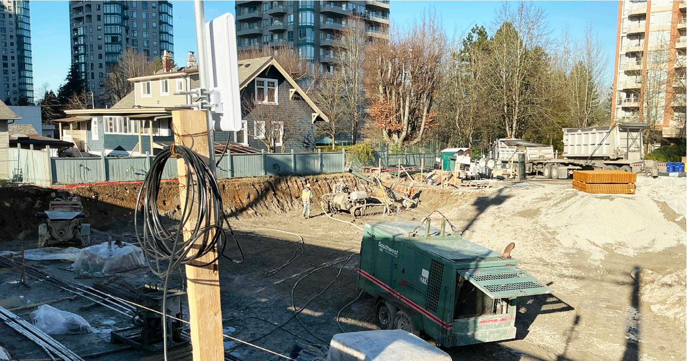
Jan 15, 2025 West Elevation. Drilling anchors for first row of shotcrete panels.
