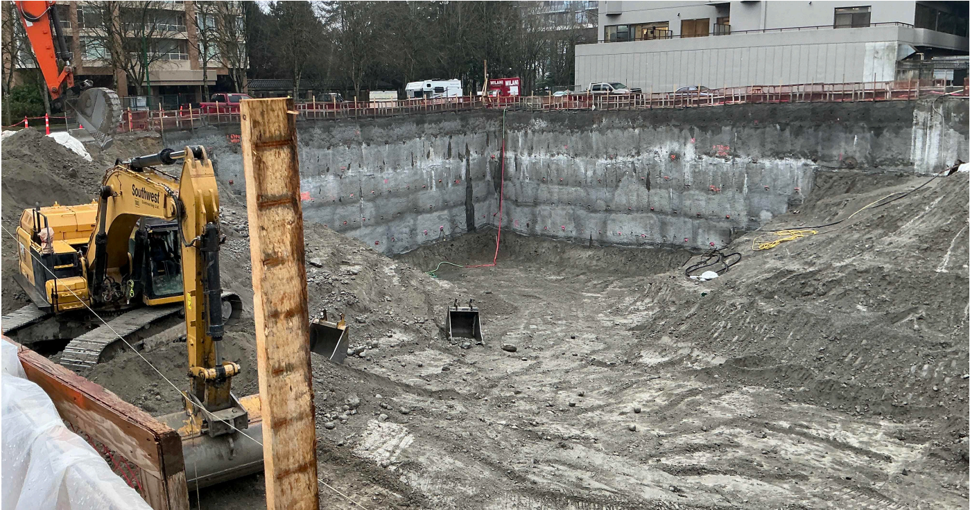
Jan 23, 2025 Excavation and shoring continues
